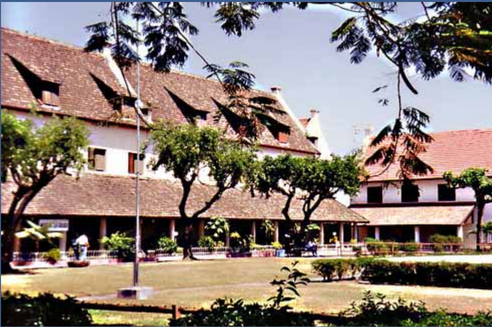
P.17 The south-west angle of Fort Rotterdam, from the gate at the sea-side to the left, photo Dirk Teeuwen 1998 The building on the left (south side) and the one on the right (west side) with the beautiful verandahs was a warehouses of the Dutch East-India Company, now Museum La Galigo. Later the building functioned as barracks on behalf of the garrison. The house in the corner (only a part of its roof is visible) served as a prison in the olden days. It is possible to pay a visit to the dungeons.
